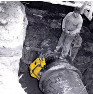
Early cutting with Trav-L-Cutter
