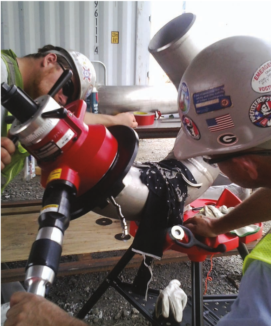
Box header beveling with SDB
