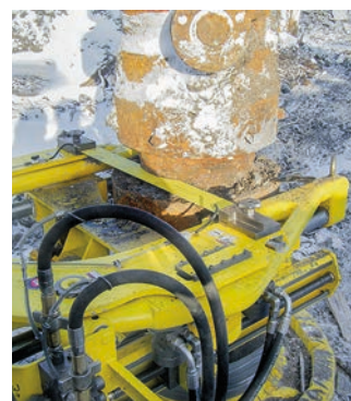
Guillotine cutting wellhead
